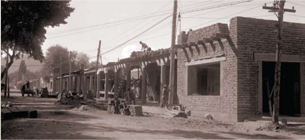
The Palace of the Governors portal under construction in 1913. Jesse Nusbaum's remodel dramatically changed the building's nineteenth century appearance into what is now referred to as Santa Fe Style. Courtesy of Photo Archives, Palace of the Governors (MNM/DCA), Neg. No. 13078.
